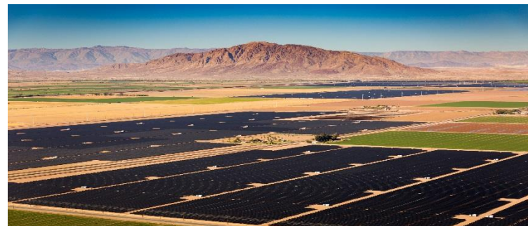
Mount Signal Solar Project in Imperial Valley
