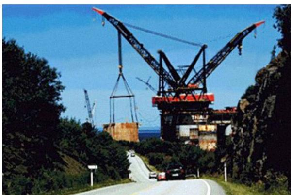
FIGURA 23: SEÇÕES DA BRENT SPAR INSTALADAS NO NOVO LOCAL PARA FORMAR A BASE DO NOVO CAIS.
